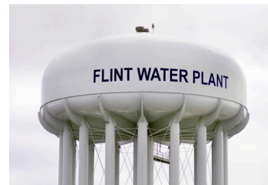
FIGURE 1: Flint, Michigan, USA, 2016 – Flint Water Plant Tank
